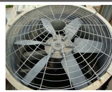
Hollow FRPs blades for cooling tower
