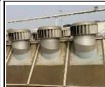
Replaced Ex fans with natural vents
