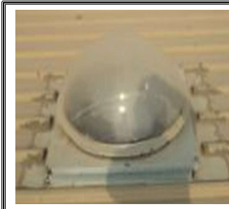
Solar Light pipes
